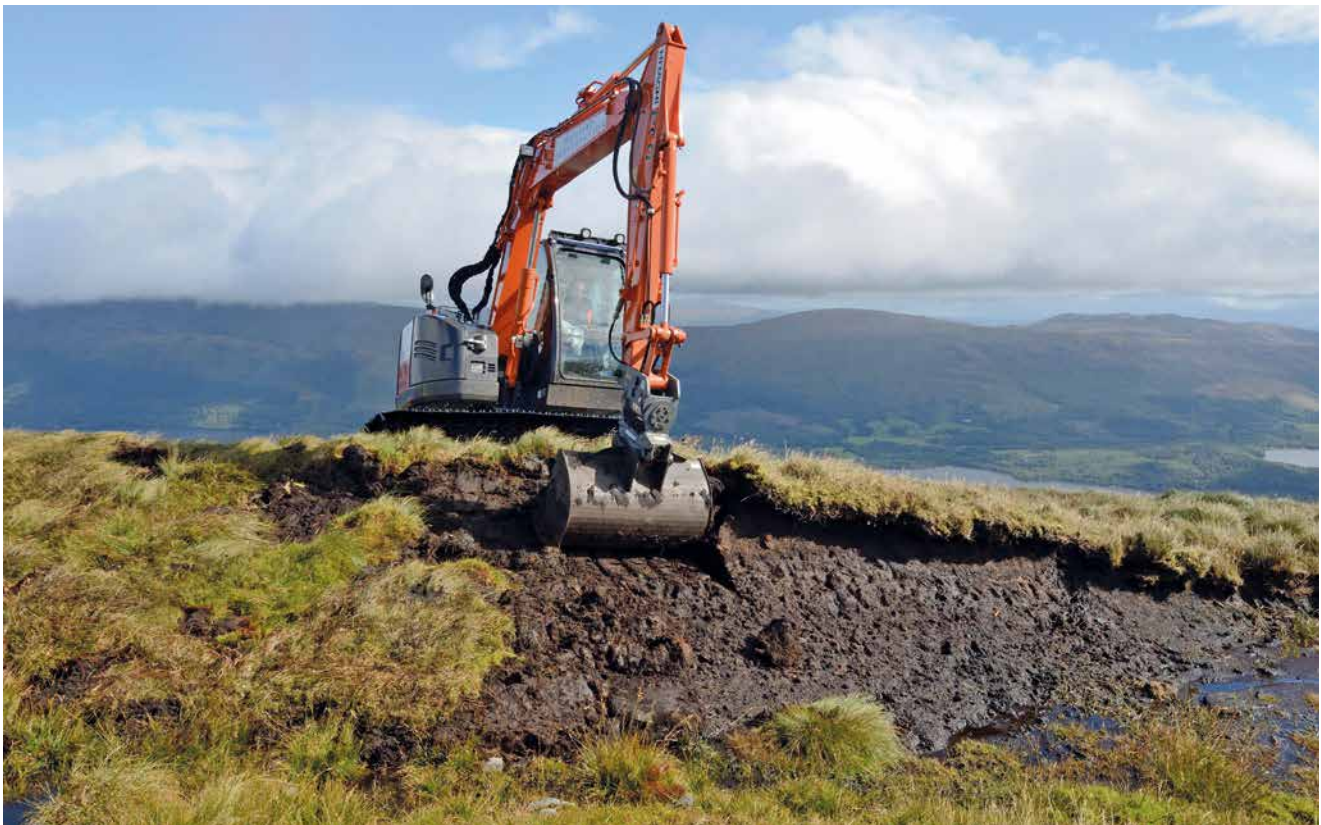
Figure 2. Digger re-profiling a peat hag. Photo credit: Peatland ACTION/NatureScot.
