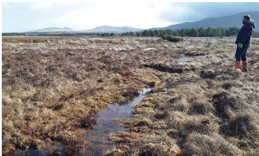
Figure 1. Blocked ditch showing peat dams and re-profiled edges, Dunlossit Estate. Photo credit: Peatland ACTION/NatureScot.
