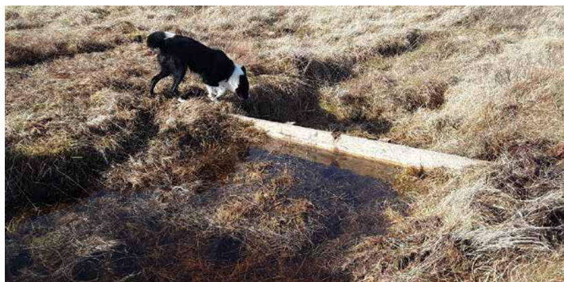
Figure 3. Wider ditch blocked with reinforced wooden dam, Dunlossit Estate. Photo credit: Peatland ACTION/NatureScot.
