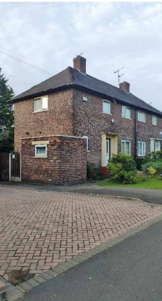
Figure 1. A typical semi-detached property with a pitched and hipped roof and open eaves.
