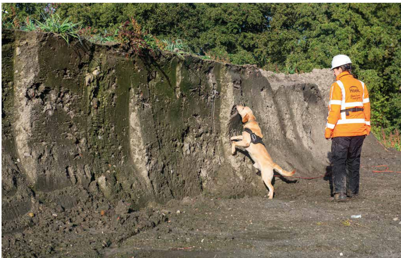
Figure 2. On the Nieuwe Kern project, controlling the deeper layers of the depot. Outside control had already taken place 3 months earlier. Photo credit: HOEK.
