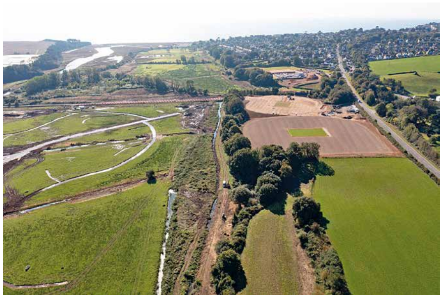
Figure 3. In Devon, the new cricket ground with two pitches (right centre) and creeks (left) that were created during the project. Photo credit: Environment Agency.
