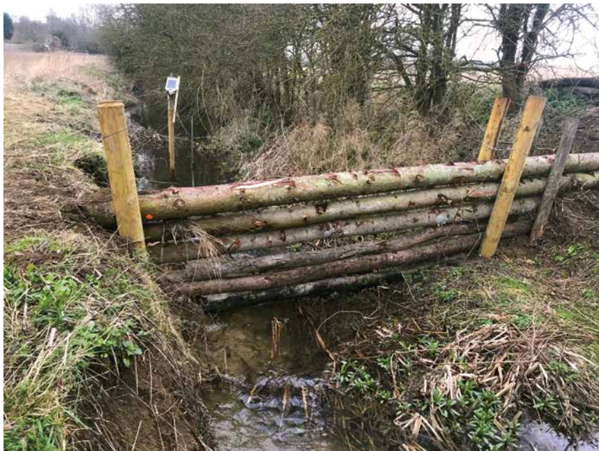
Figure 2. Leaky dam holding back the flow on Finchingfield Brook. Photo credit: Spains Hall Estate.
