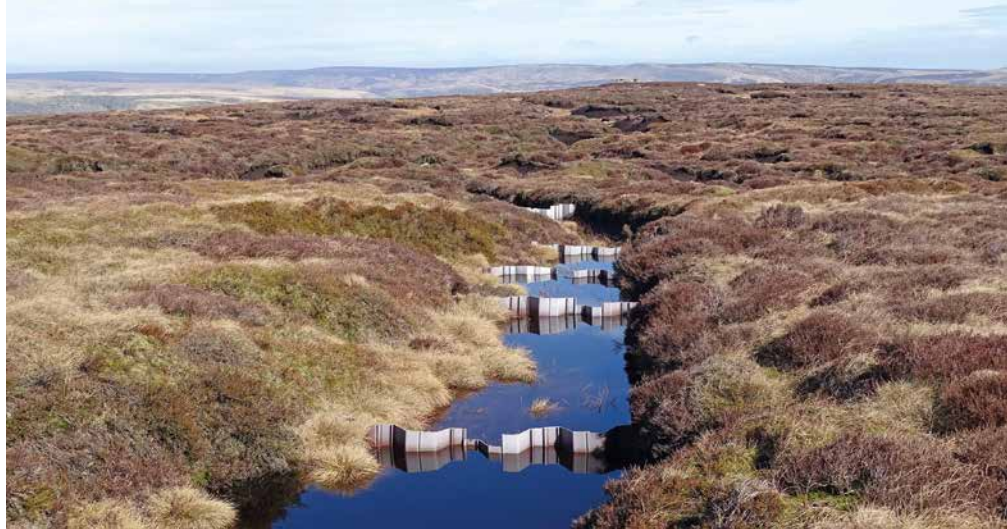
Recycled plastic piling used to block a gully to rewet blanket peat, Peak District. Photo credit: Penny Anderson.
