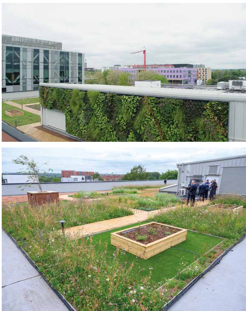
Figure 1. IGNITION Nature-based Solutions Living Lab at the University of Salford, with a green roof and a green wall. Photo credit: The IGNITION Project.
