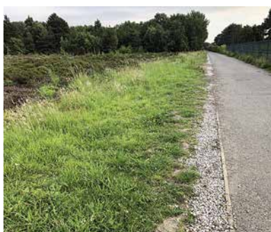
Figure 3. Damage to a Sefton dune heath through path extension and the application of lime chippings (2020). Photo credit: Josh Styles.
