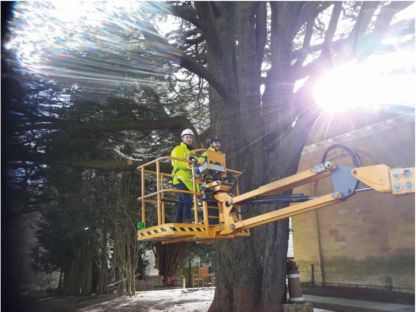
Figure 3. Installing bat boxes to provide alternative roosts for bats to use. Photo credit: Laura Holmes.
