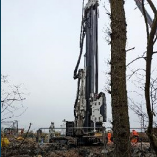
Noise measurement of Auger piling
