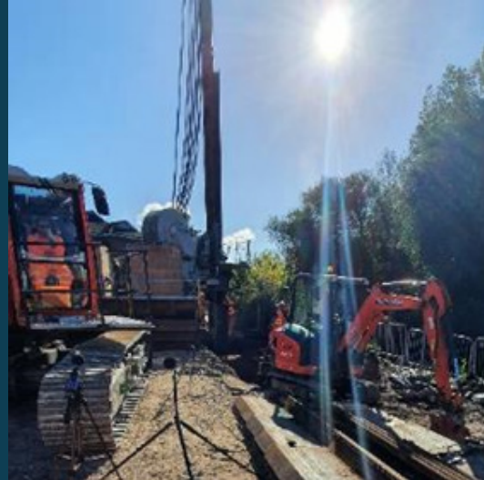
Noise measurement of Giken piling
