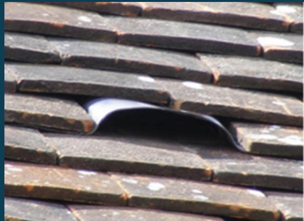
Bat slate in position (neat and unobtrusive).
