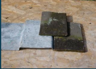
How the completed Bat-slate will fit amongst the tiles.
