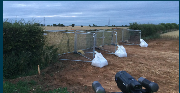
Rear face of panels showing triangular bracing (Photo: A. Logan).
