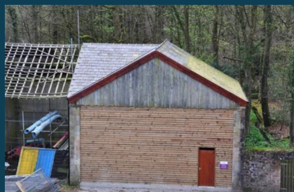
Detail of the compensation building (bat barn)
