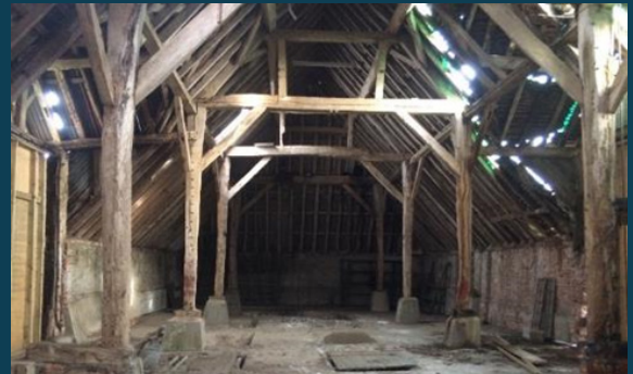
Northern part of the barn prior to screen installation
