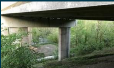
View of PNV Viaduct, looking east.
