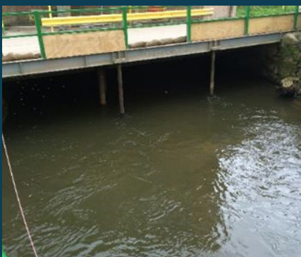
Western end of culvert
