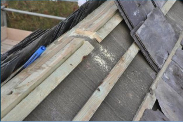
Cut battens for access under the ridge (P. Waring)
