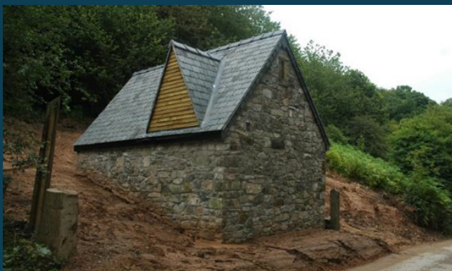
Replacement roost July 2011 (south-western elevation)
