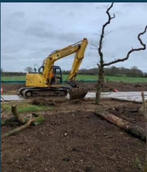
Once secured, machines can work safely in close proximity
