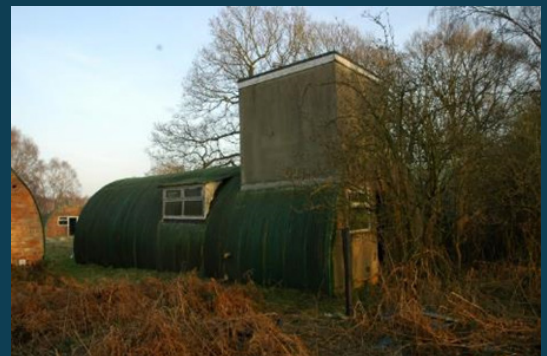
Building prior to start of works
