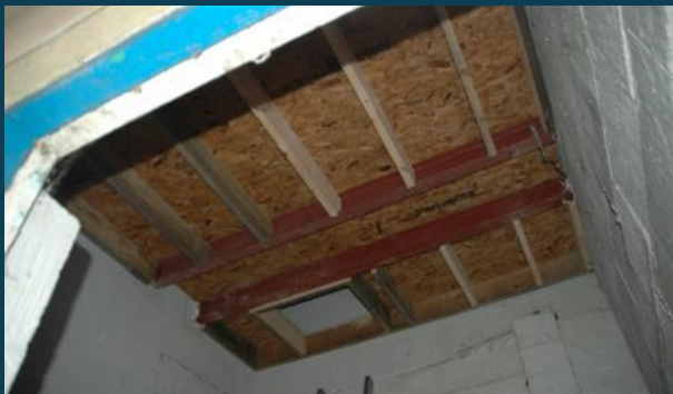
Internal – ceiling inserted 1.5 m below flat roof
