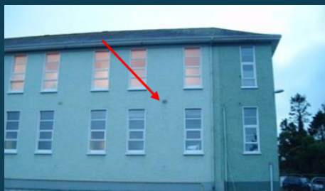
Ventilation grille used by soprano pipistrelles
