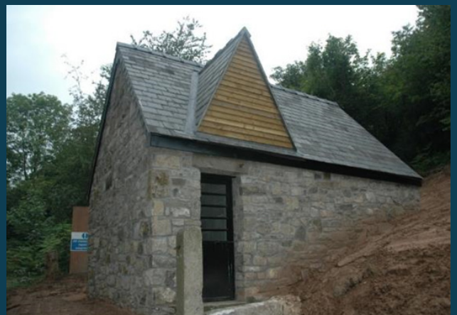
Replacement roost July 2011 (south-eastern elevation). Located adjacent to quarry access road on woodland edge set into a steeply sloping bank, 150 m from the original roost. By setting it into the bank, it enabled the northern gable end to be partially buried and ensured suitably cool and humid conditions for transitional and hibernation use.
