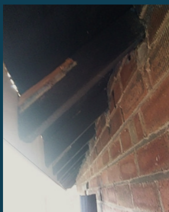
Eaves of completed roof
