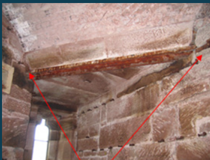
Roost entrance in stone which provides access behind the lintel
