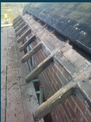
Stripped wall plate
