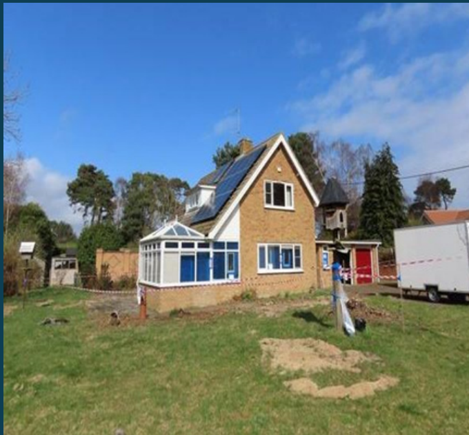
Overview of the building
