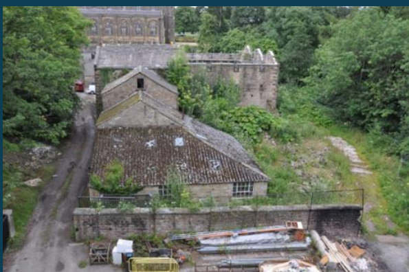
Overview of the original bat roosts, prior to deconstruction
