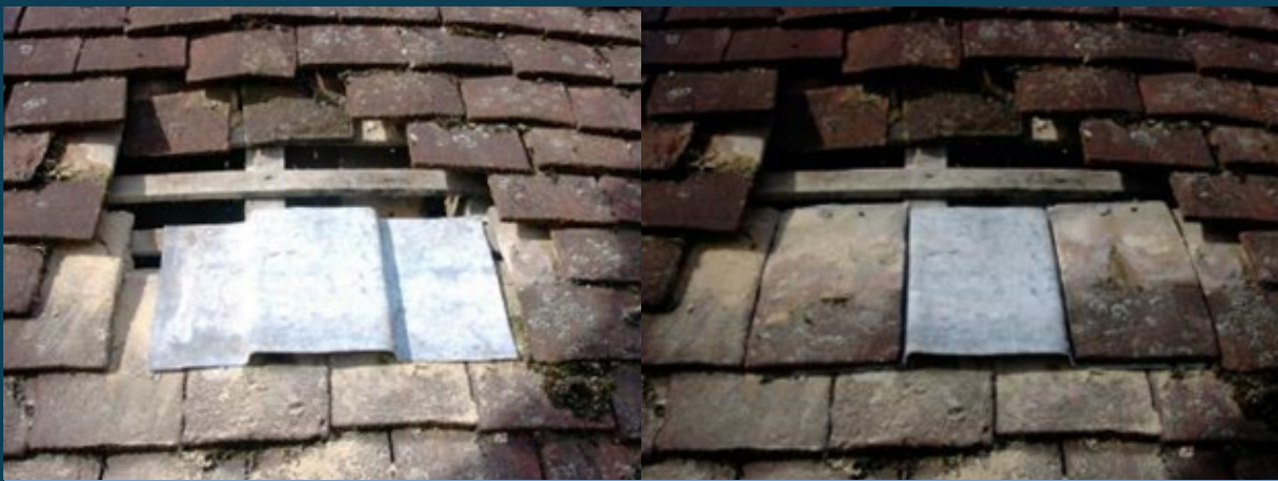
The Bat-slate is fitted alongside a rafter, allowing bats to land and crawl out. On a new or re-furbished roof, a hole will need to be established in the felt. The Bat-slate shown here is fitted so that a whole tile will fit alongside it. Where this isn't possible, the tile(s) will need to be cut. The Bat-slate is nailed (x2) to the batten and the tiles refitted around it.
