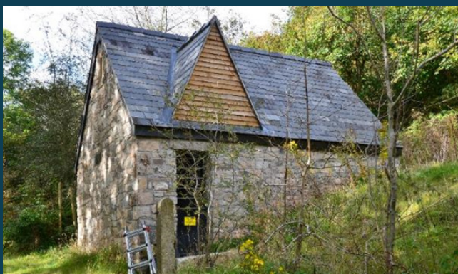
Replacement roost July 2014 (South-eastern elevation), three years later
