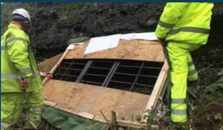
Partial closure of the adit entrance
