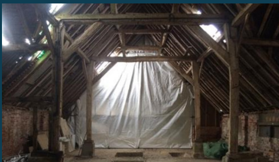
Screening in place
