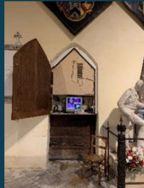
The interior artificial roost installed, with false door open
