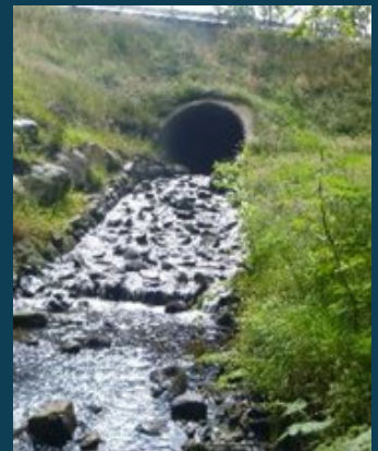
The culvert with stream flowing through
