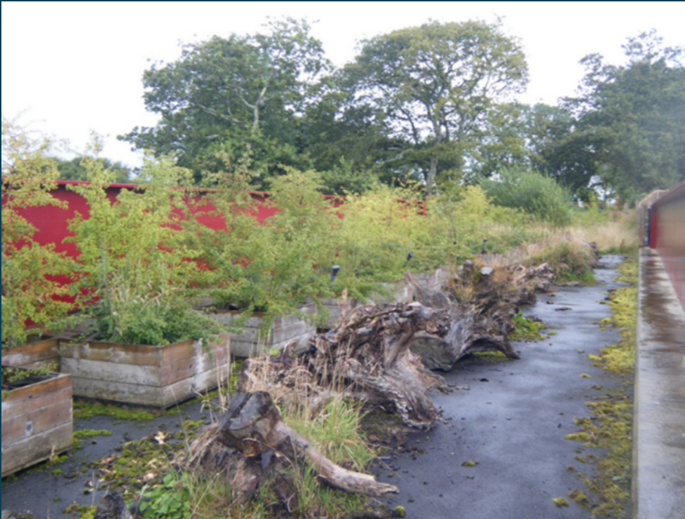
Planters and tree stumps on bridge deck
