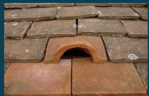
Bat access tile installed within the farmhouse roof
