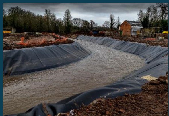
Diversion of river in place
