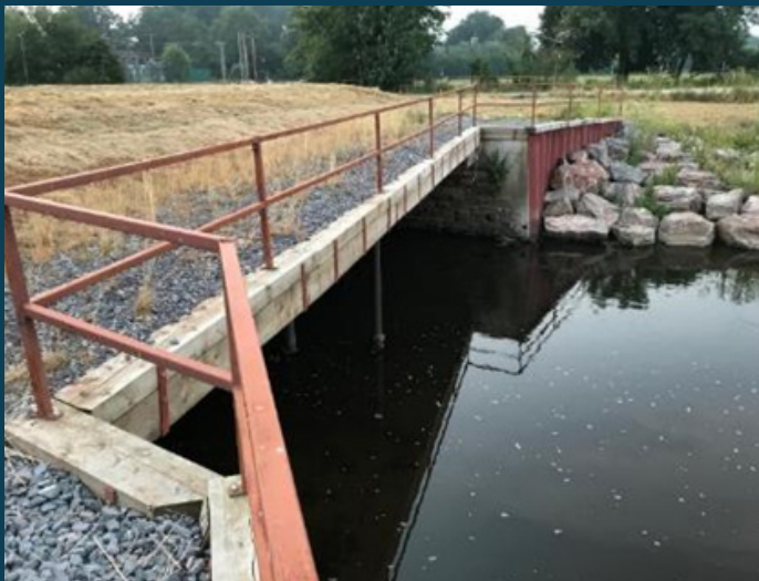
Retained section of the culvert used by the colony
