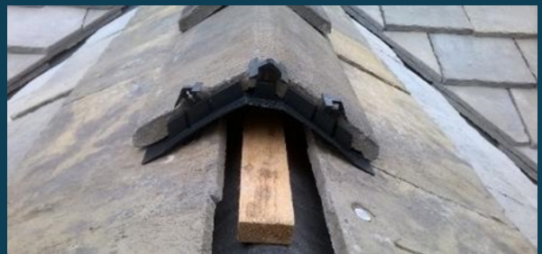
Ridge tiles showing tile and plastic union installed over batten
