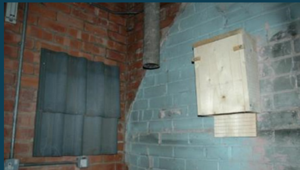
Bat boxes and hanging tiles were added to the internal walls – although these do not appear to have been used
