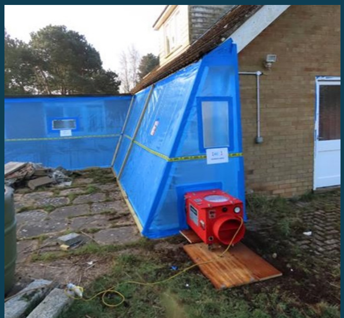
Negative Pressure extractor pump and filter
