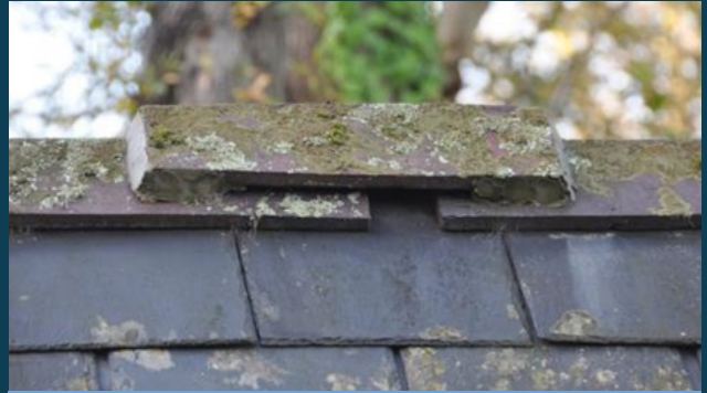
Access to wet-ridge site (P. Waring)
