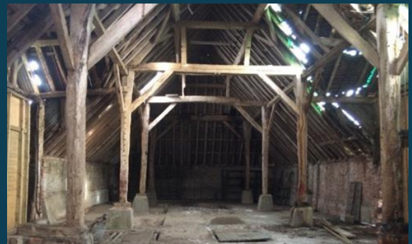
Northern part of the barn prior to screen installation
