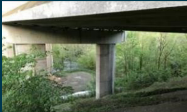
View of PNV Viaduct, looking east.
