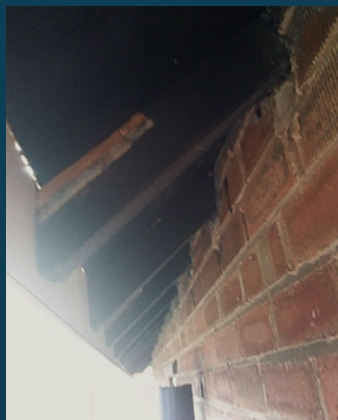
Eaves of completed roof
