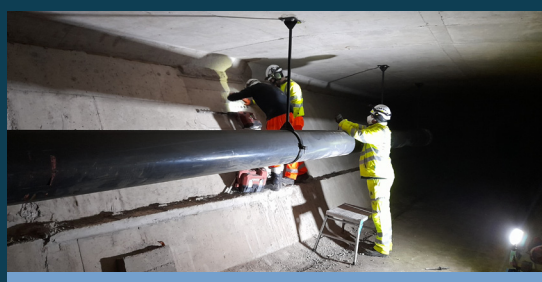
Core drilling in progress: note lighting and human ear defenders
