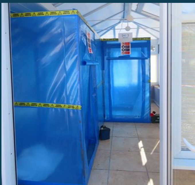
Overview of the building
