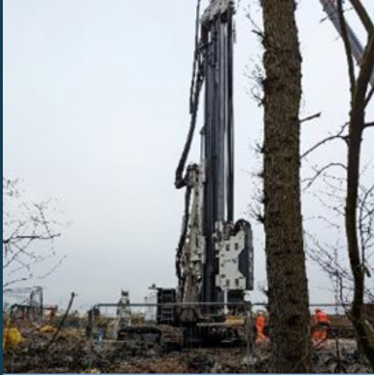
Noise measurement of Auger piling
