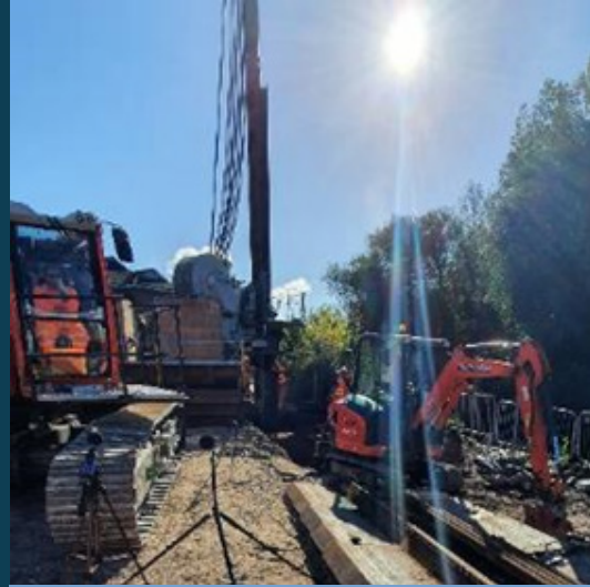
Noise measurement of Giken piling
