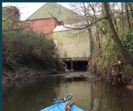
Eastern end of culvert
