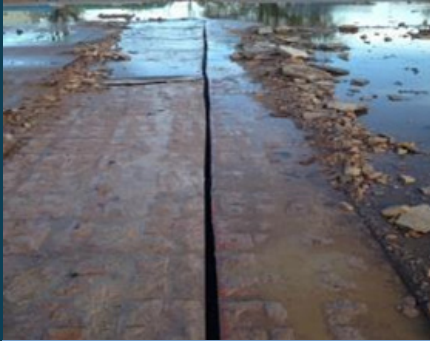
Diamond cut through culvert slab
