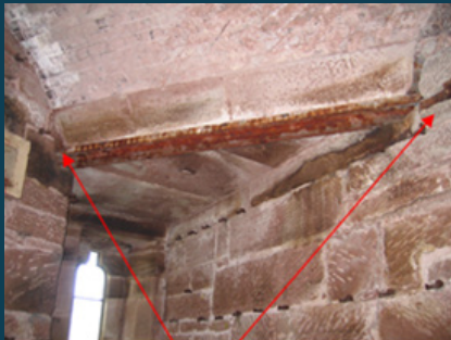
Roost entrance in stone which provides access behind the lintel
