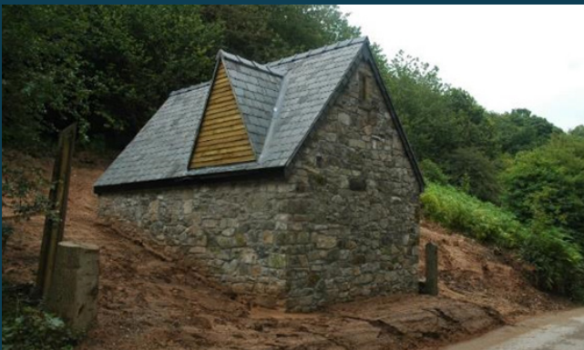
Replacement roost July 2011 (south-western elevation)
