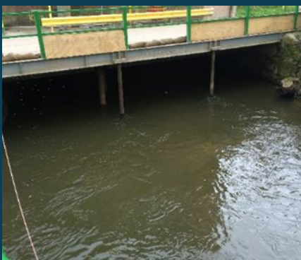
Western end of culvert
