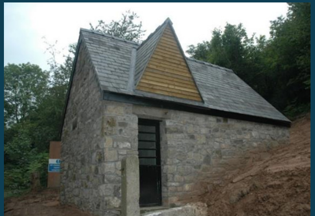
Replacement roost July 2011 (south-eastern elevation). Located adjacent to quarry access road on woodland edge set into a steeply sloping bank, 150 m from the original roost. By setting it into the bank, it enabled the northern gable end to be partially buried and ensured suitably cool and humid conditions for transitional and hibernation use.
