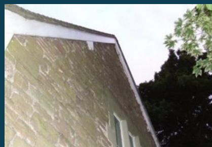
Bat access point at gable apex
