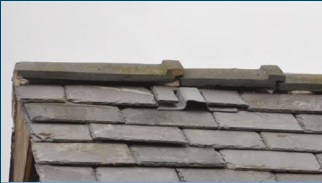
Ridge access feature (P. Waring)
