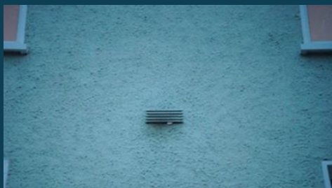
The grille allowed bats to enter the wall cavity
