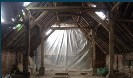
Screening in place
