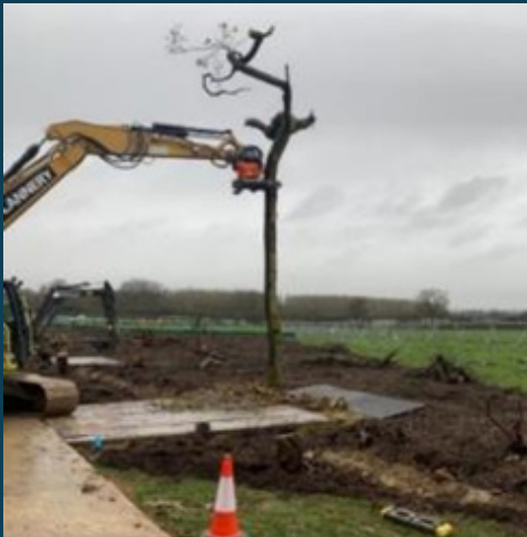
The monolith is lifted into position
