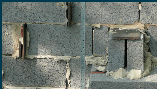
No access to these same cavities was provided from the outside, to avoid draughts. A number of other external roosting features were provided, including accessible barge boards at gable ends, and lead slips within roof coverings.
