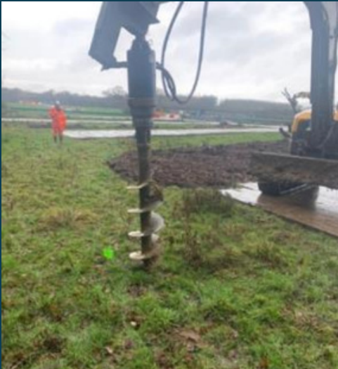
An auger attached to the excavator prepares the pit
