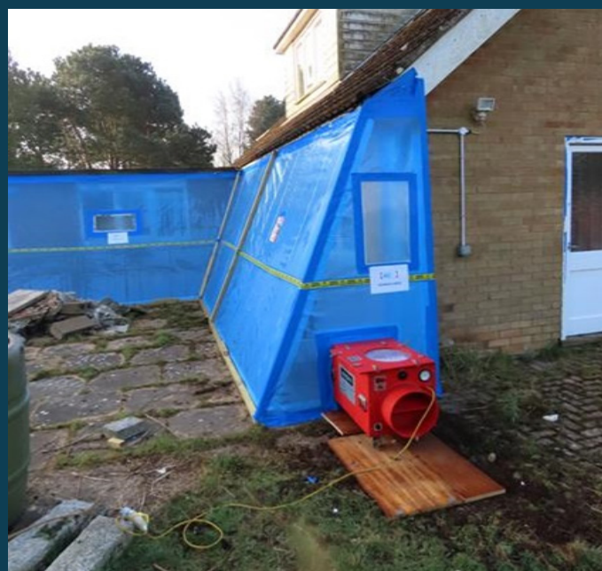
Negative Pressure extractor pump and filter
