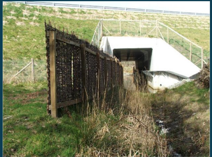
Culvert with hurdle fencing guide
