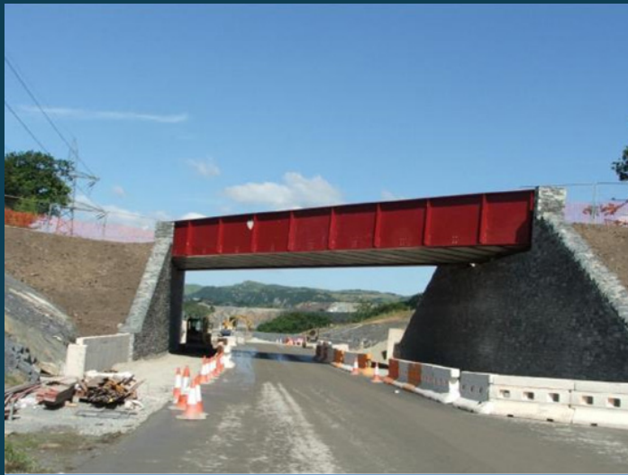
Bridge crossing during construction
