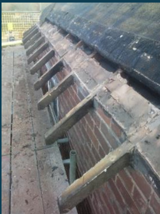
Stripped wall plate
