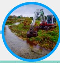
restore the gravel stream-bed, using material similar to that found in local intact river beds (avoid using graded and outsized material)
