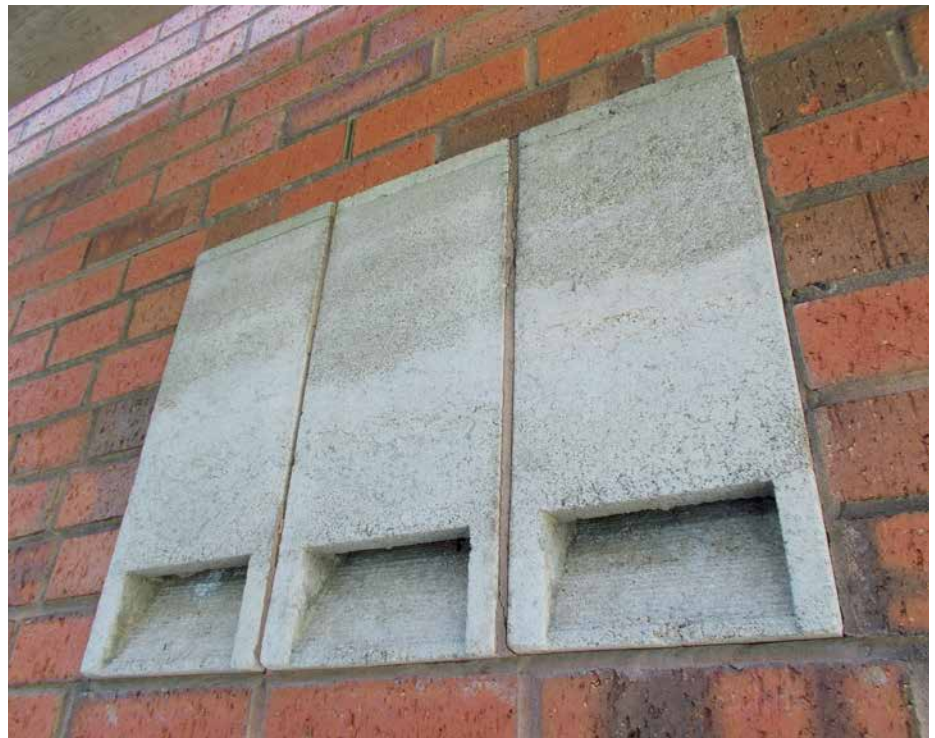
Bat tubes built into brick wall. Photo credit Andrew Ross.
