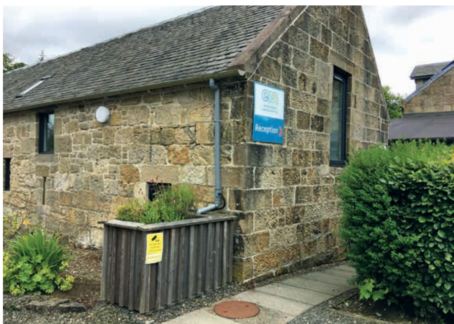
Planter box rain garden installed at CSGN's offices, planted with a range of native wildflowers and herbs that can cope with periods of wet and dry. © CSGNT.
