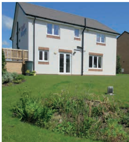
Figure 2. In-ground raingarden installed in a Taylor Wimpey show-home. Positioned at the lowest part of the garden, it collects and uses the rainwater, helping to drain the rest of the garden. © CSGNT.
