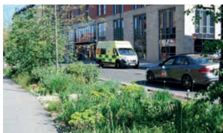
SuDS draining the highway in Sheffield as part of their Grey to Green project.
