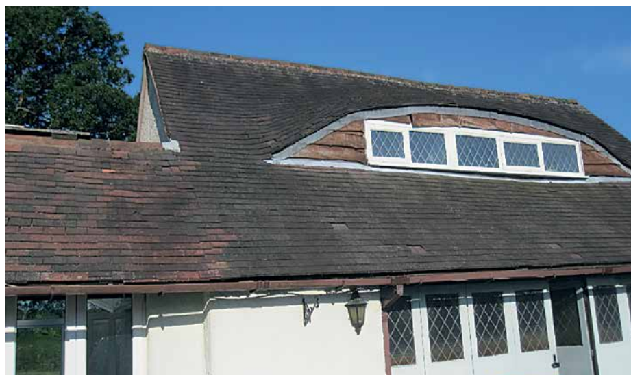
This house, located in an area of excellent bat foraging habitat, with slipped/missing roof tiles and gaps beneath weatherboarding/lead flashing leading to voids behind, was deemed to have "negligible bat potential" by a surveyor. Photo credit Lisa Kerslake.
