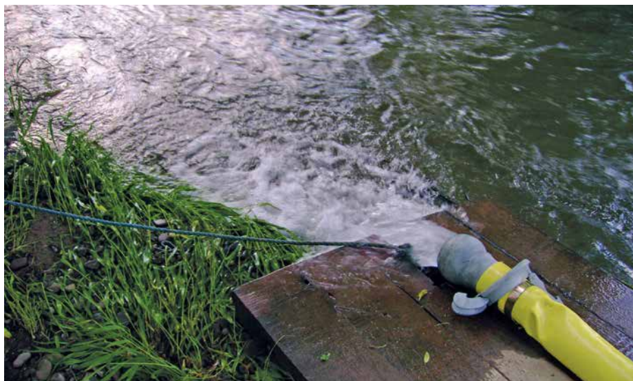
Pumping clean water back to watercourse whilst avoiding scour of channel bed.
