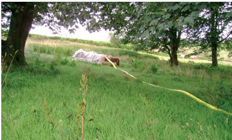
Intercepting rainfall and pumping upslope to adjacent grassland to protect watercourse.
