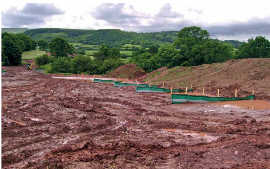
Extensive deployment of silt fencing and other preventative measures being overtopped by high rainfall event.
