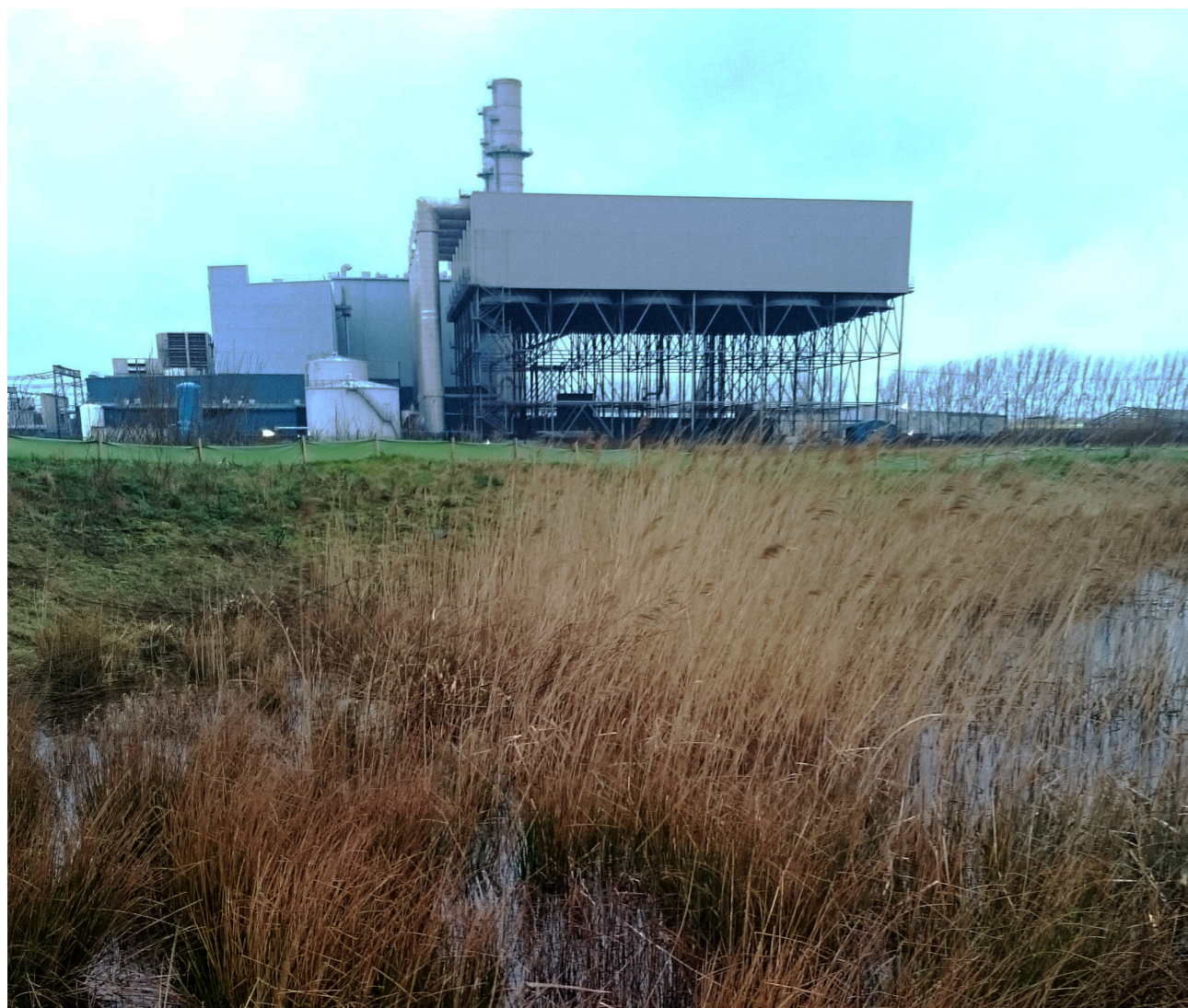
Ecological mitigation area adjacent to gas-fired power station. Photo credit: Philip Peterson.
