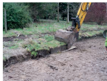
Figure 4. Modified method, placing turf on to plywood to reduce breakage, November 2014 (Right)
