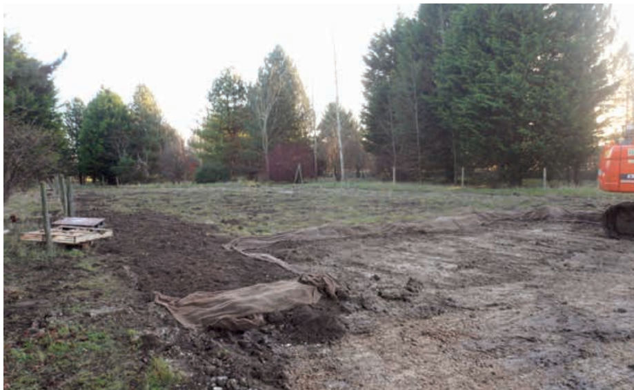
Figure 2. Hessian used to protect exposed edges of turves at receptor site in November 2014.
