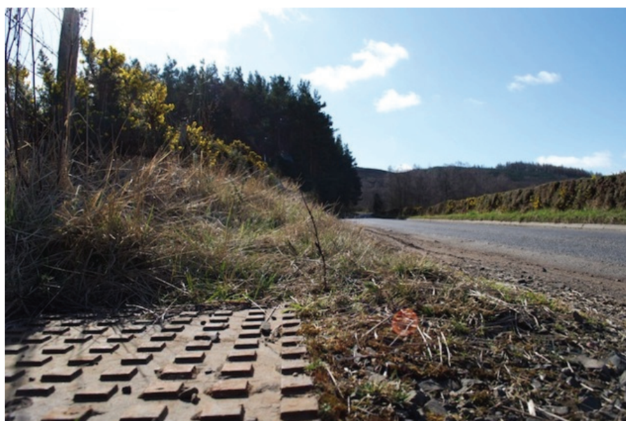
Figure 14. Road verge hazard to cutting machinery
