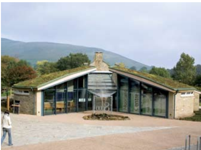
Peak District National Park's Moorland Centre reflects its upland setting. It has a living turf roof for insulation and is heated by a ground source heat pump
