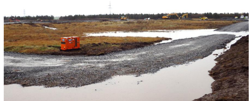
Site in 2015 during early earth works.
