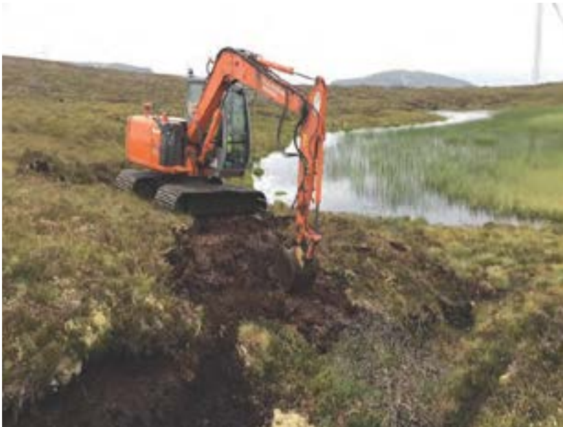
Figure 23.1 Restoration works (before)
