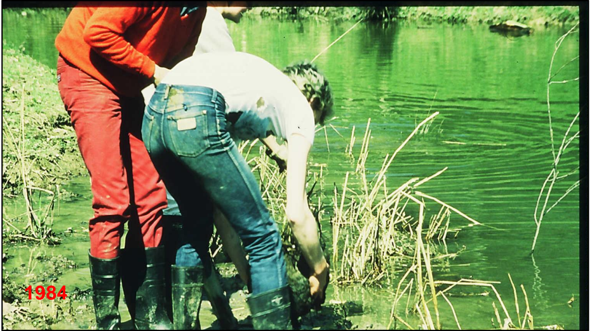
The rhizomes of common reed were planted into the clay bottom in shallow areas.
