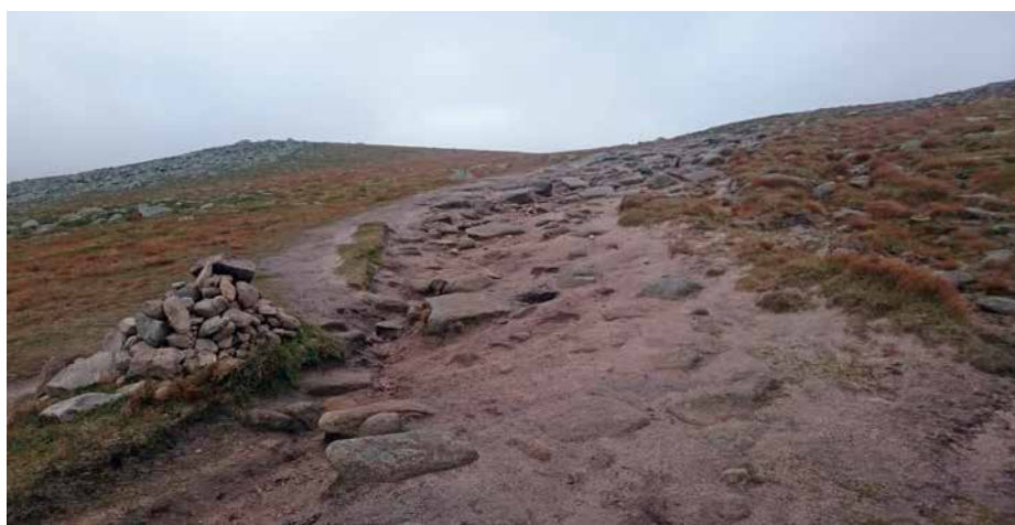
Lochnagar in the Cairngorms, before restoration – path eroded and braided to 5 m wide.
