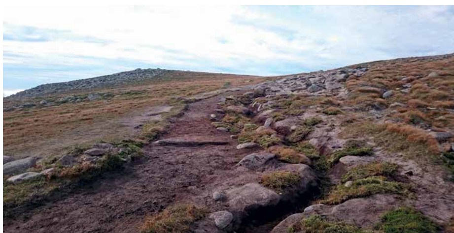
Lochnagar after restoration – path defined at 1.2 m wide, drainage installed and landscaped to the surrounding site.
