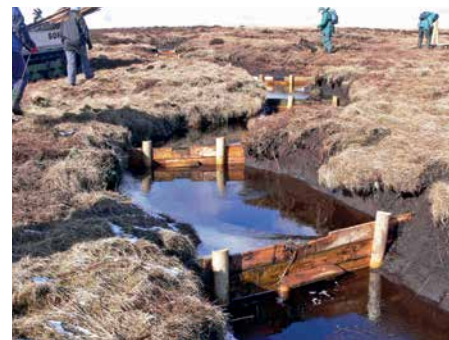
Wooden dams installed on Marsden Estate (South Pennines) by the National Trust.
