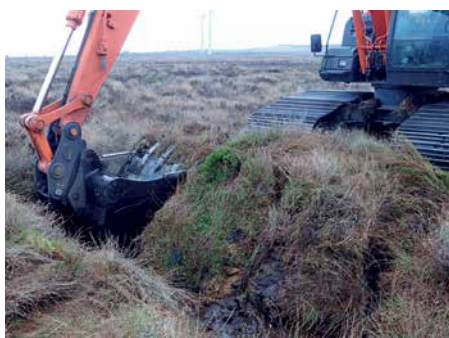
Figure 9. An excavator using its bucket to compress the thrust peat material to form an elevated ridge, with vegetation remaining on the surface.
