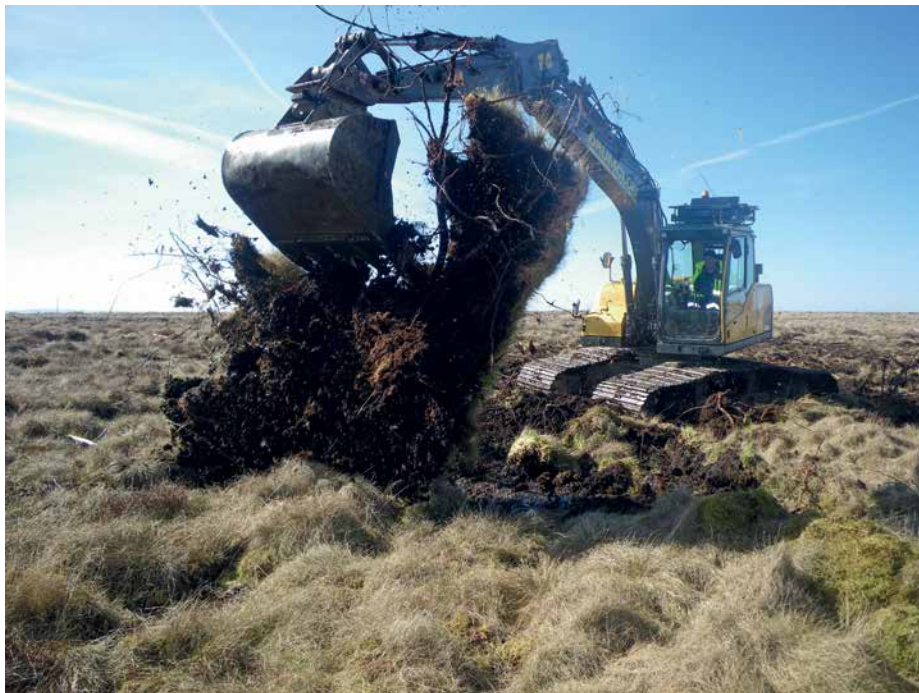
Figure 2. An excavator turning over a stump and root plate using the ground smoothing method.
