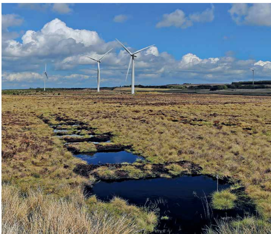
Figure 10. A finished row of wave dams holding water along a drain.
