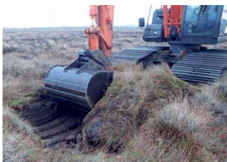
Figure 8. An excavator using its bucket to pull a second cube of peat towards itself. Note the first cube of peat that has already been thrust towards the machine to the right of the bucket.
