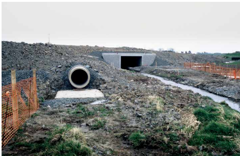
Mitigation involving the creation of a fauna passage and culvert. © Adam Grogan.
