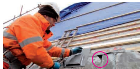
The roof of this chapel had multiple roosts between slates and boards with access not always obvious. Note the felt flap nailed to lath top side of replacement roost to prevent bats being able to pass over lath and come in contact with the BRM. This was an extra precaution.
