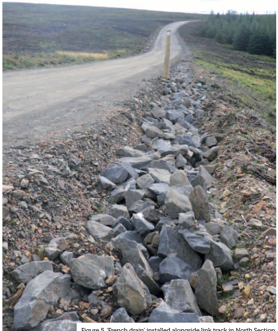
Figure 5. 'French drain' installed alongside link track in North Section.
