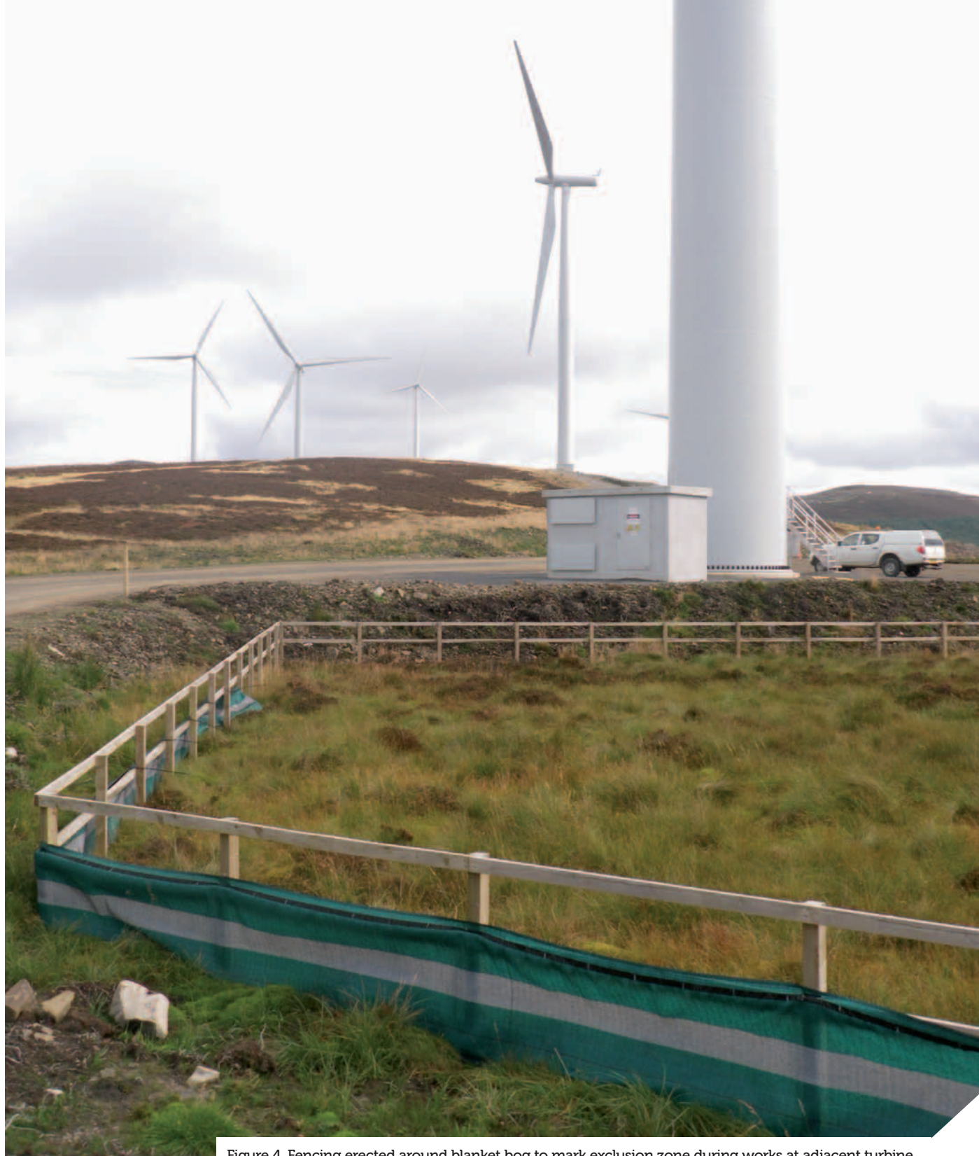
Figure 4. Fencing erected around blanket bog to mark exclusion zone during works at adjacent turbine.
