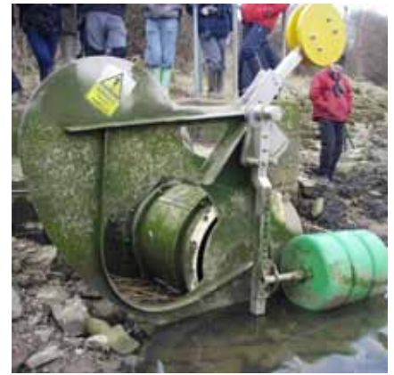
Figure 4. The self-regulating tidegate
