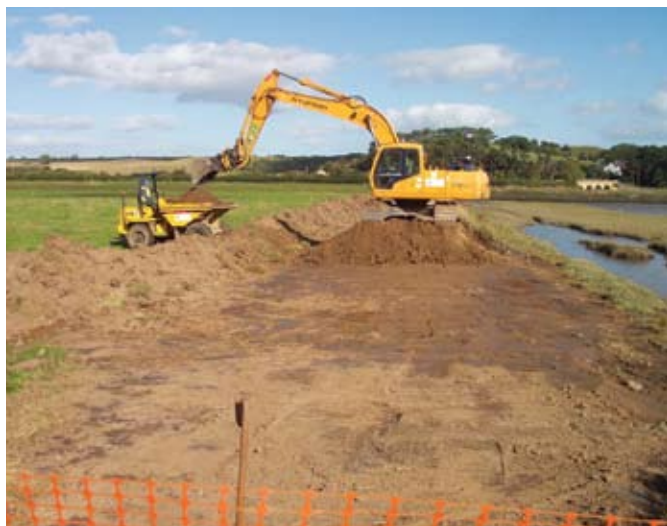
Machine works on the Alnmouth saltmarsh floodbank
