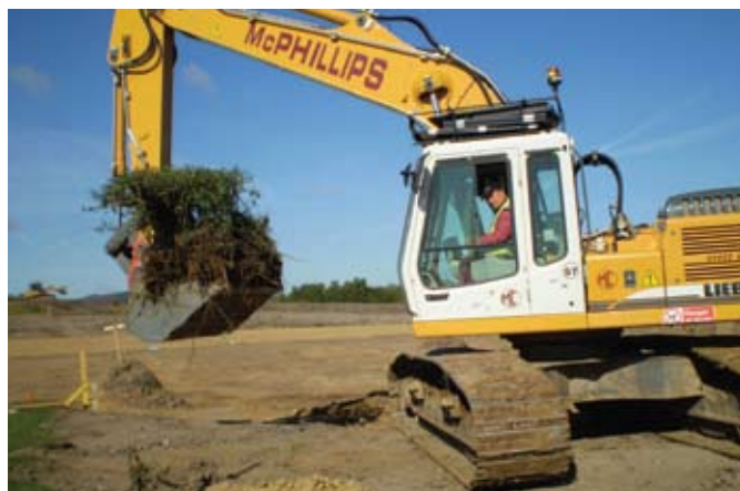
Photo D. Moving a section of hedgerow in September prior to earthworks operations
