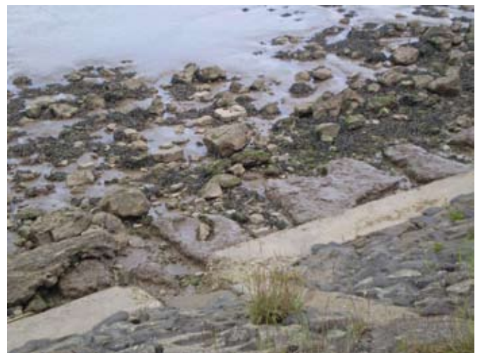
Photograph 2. Foreshore erosion in front of the sea wall at North Killingholme, North Lincolnshire. This illustrates the loss of fine muddy sediment and exposure of harder consolidated sediments.
