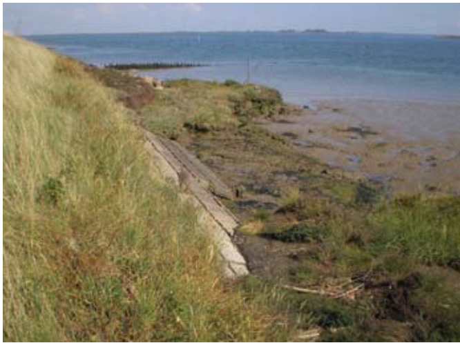
Photograph 3. Saltmarsh erosion exposing the toe of the sea wall at Wallasea Island, Crouch and Roach Estuary, Essex. This photograph shows classic coastal squeeze features: cliffed saltmarshes, lowered mudflats and undermining of sea walls.
