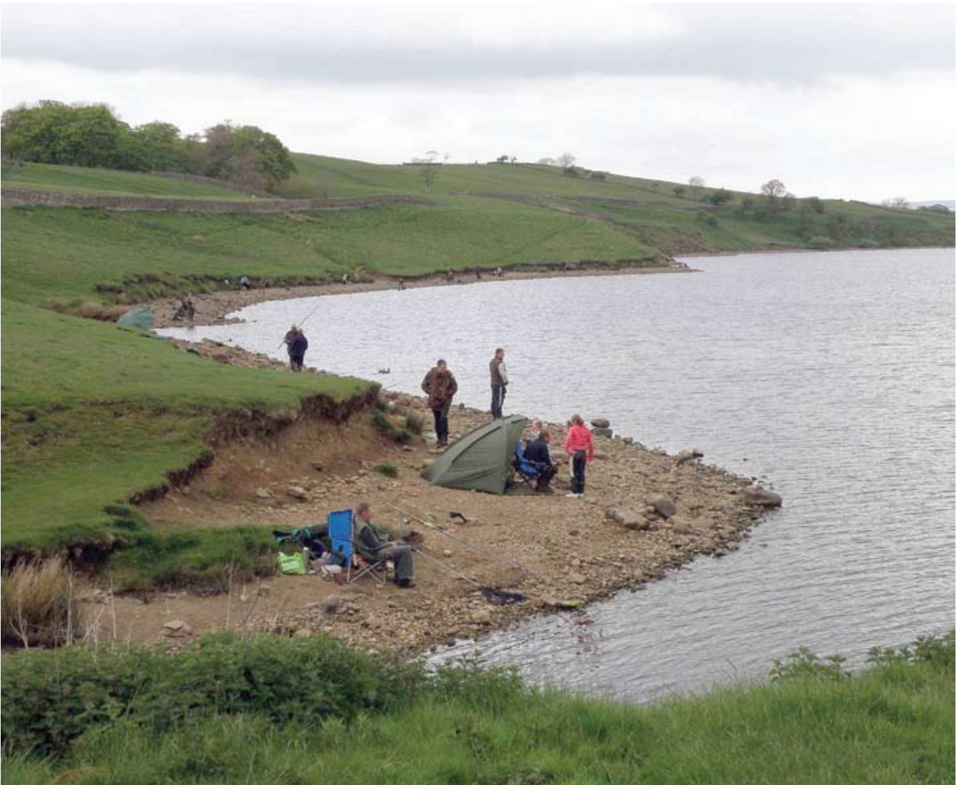
Photograph 1. Foreshore erosion on the Grassholme Reservoir (NW Yorks). Note that the erosion cliff comprises material of varying diameter, primarily fine grains. The foreshore below the erosion cliff is, however, predominantly coarser material.
