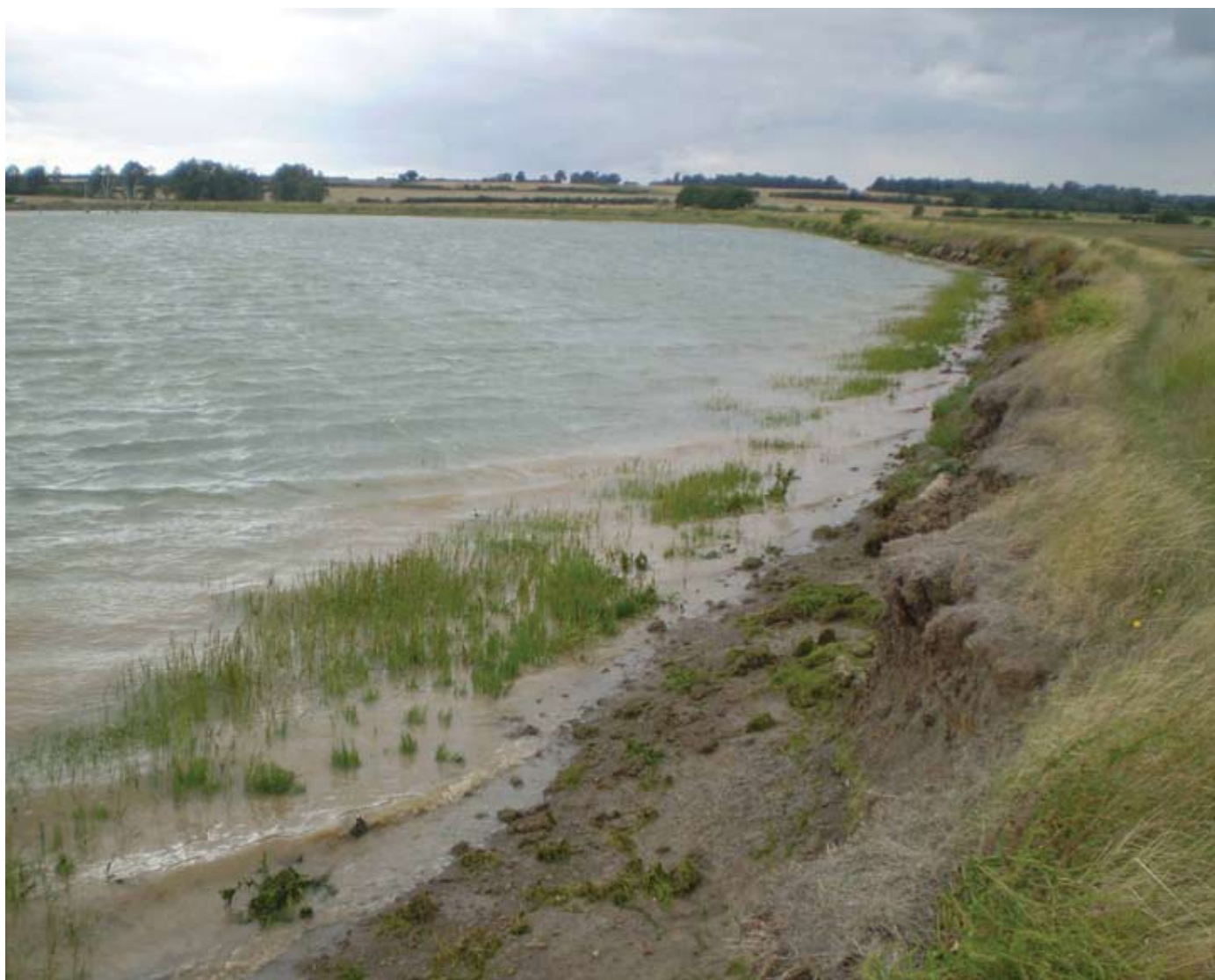
Photograph 2. Tollesbury managed realignment site. Here former sea walls on the inside of the realignment are eroding through wind-driven wave activity. Evidence of sediment mobilisation is clear through the band of muddy water adjacent to the shoreline. This mobilised sediment will be drawn offshore as the tide ebbs, after which it will be dispersed and may settle sub-tidally.
