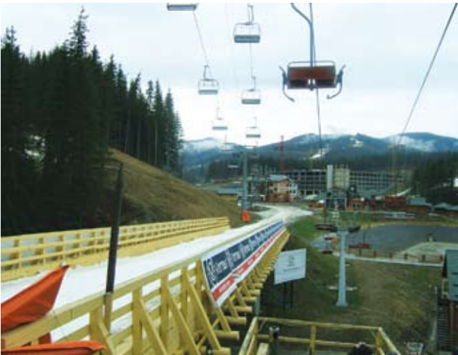
Development work in Bukovel, Ukraine Photo: Wilf Fenten
