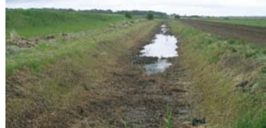
Water vole mitigation: vegetation removal and dewatering of soke dyke
