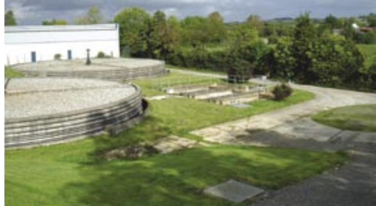
Nenagh Waste Water Treatment Works - in the heavily designated Shannon catchment
