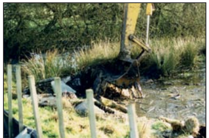
Plate 5. Desilting and deepening being carefully undertaken on pond 6 during a cold day in mid-winter 2002/2003.
