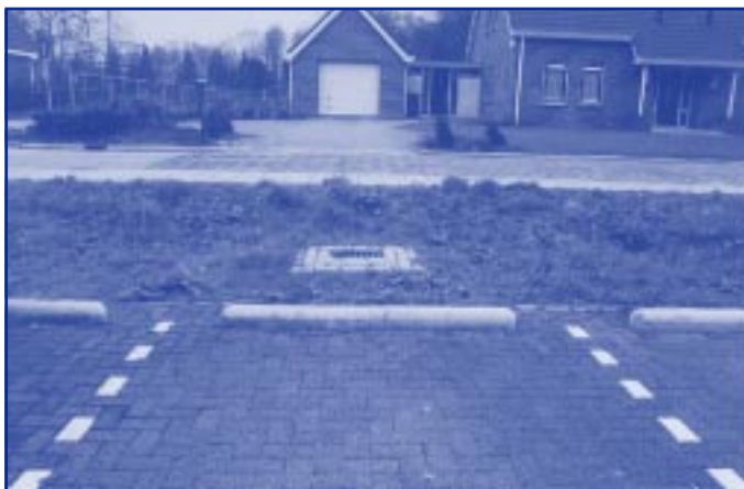
Swale just after Construction
