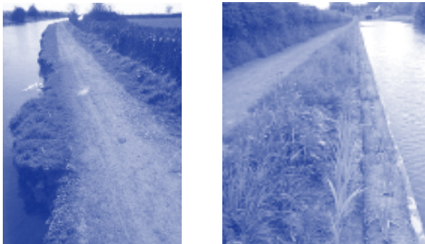
Figure 7: Photographs taken before and 6 months after the construction of the castellated permanent moorings.
