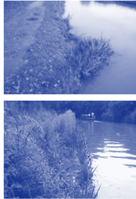
Figure 5: Photographs taken before and 6 months after the construction of a hazel faggot vegetation shelf.
