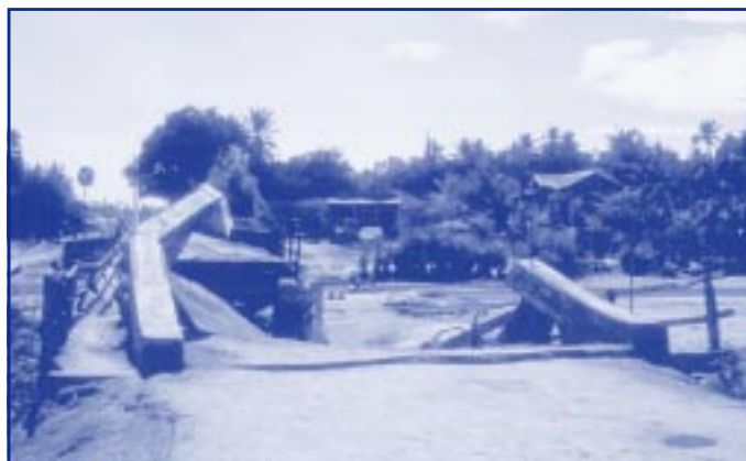
Figure 1 : Shelled bridge, Highway 6, Kampong Chamm, Cambodia.
